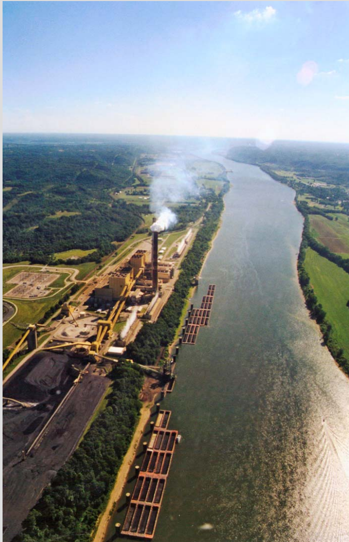
Ohio River coal power plant
