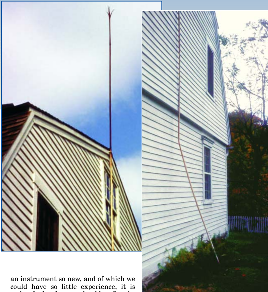
Figure 5. An 18th-century house with a lightning rod of Franklin's 1762 design. The thick, continuous rod can carry tens of kiloamperes of current to ground without harming the house or its foundation.
